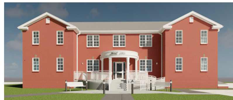
Moor Hall (above) is currently being renovated to become the Beaufort Campus' new admissions and enrollment HUB. Original to the Mather School, the historic building has housed classrooms and also served as an administration building, a science laboratory, a library and a bookstore since it was built in 1939.
